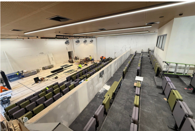
Theatre seating, flooring, and ceiling installed. Wall finishes and glass balustrading will complete the theatre works in the coming weeks.
