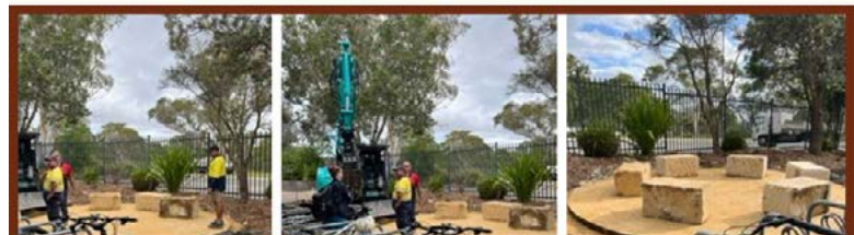
KMHS Yarning Circle Photos above show construction and landscaping in progress at the school.
